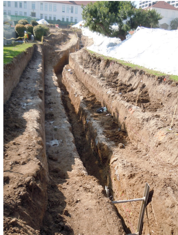
Fig. 4: One of the exploratory trenches excavated to expose and map the faults that were mapped through the BHHS, part of which is seen at the top of the photo. Each bench is about 1.3 m in height; shoring was used where space did not permit benching. No faults were found in this trench.
